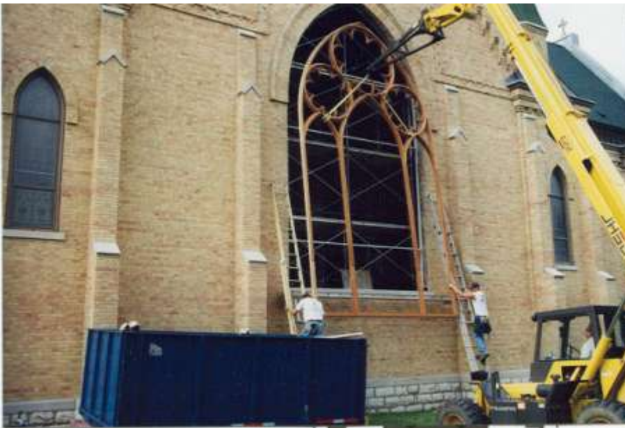
Left:: Installation of window tracery 2001. Installation cost for Nativity and Ascension Windows, $250,000
