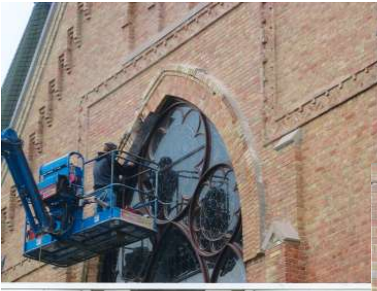
Repair in progress. November 2009
