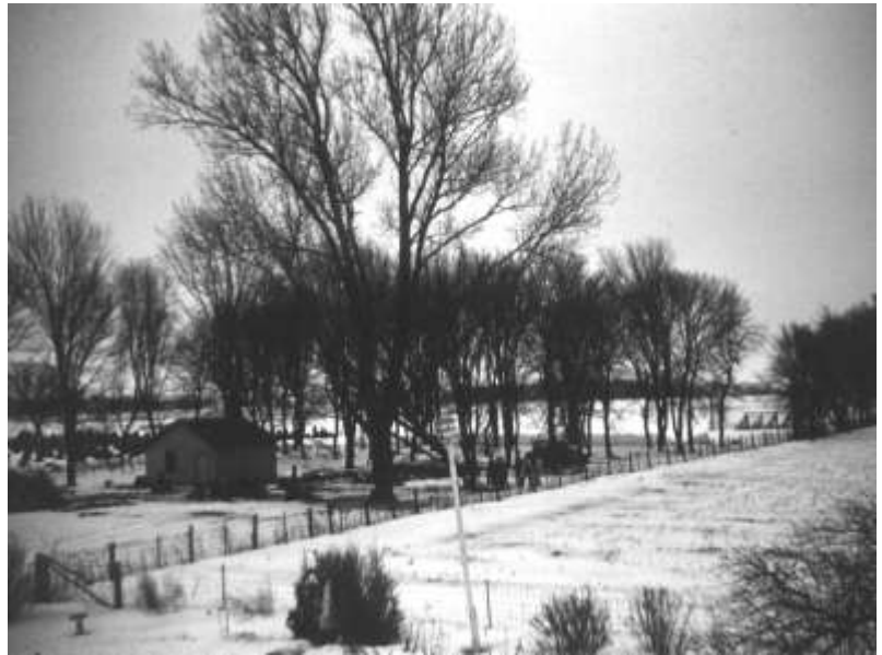
Parish Park before groundbreaking. Huge Poplar tree in foreground was cut down by a two man chain saw manned by Armond Wass @ Sons. Farmers from the parish spent the winter hours to clear the park for the new school. Little white building served as a kitchen for summer picnics
