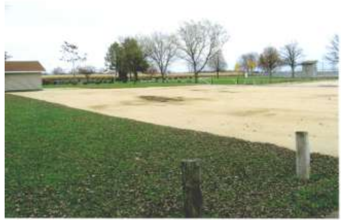
New parking lot
