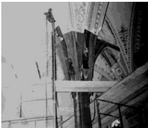
Church interior reconstruction 1958
